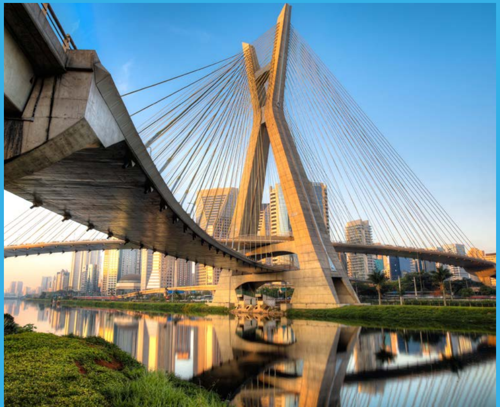
Estaiada Bridge, Sao Paulo, Brazil
